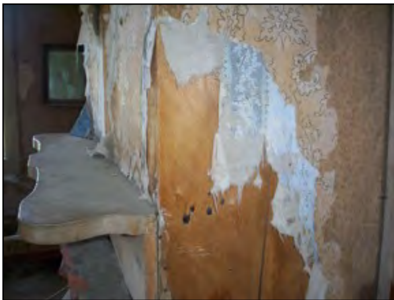
Photo 8: Miller House wall detail. Wood probably from Mono Mills topped by a gauze cloth and two cloth wall coverings. Note the cut and wire nails.
